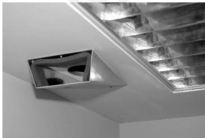
Fig. 6. Directional beacon mounted on top of ceiling and reproducing sound through holes. Aluminum bracket gives loudspeaker its directional properties.
