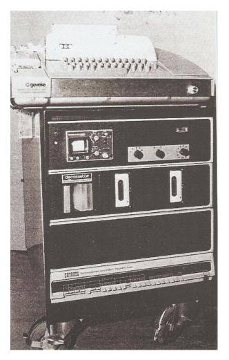
Figure 1. STIDAS I (STI Device using Artificial Signals) device based on a PDP-11/10 computer and custom analog hardware (1971).
